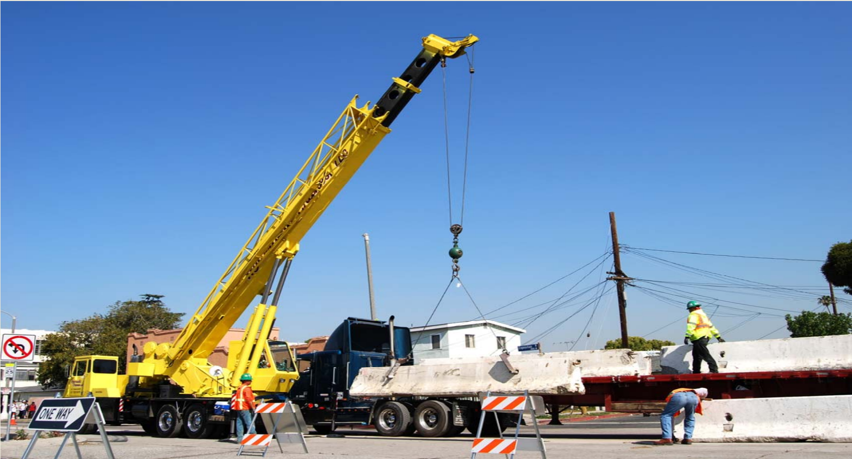
K Rail Installation from Vermont to 7 th Avenue
